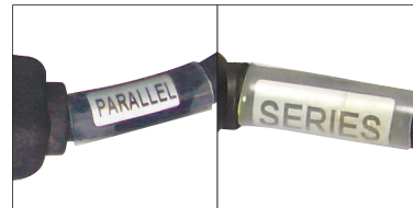
Parallel / Series sticker mark with transparent heat-shrink sleeve identify the wirings clearly.
