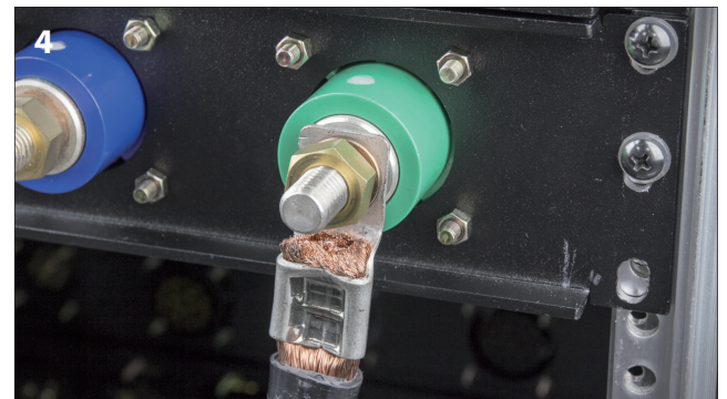
Refit the washer and nut onto the threaded post, then tighten to max. of 12N/m
