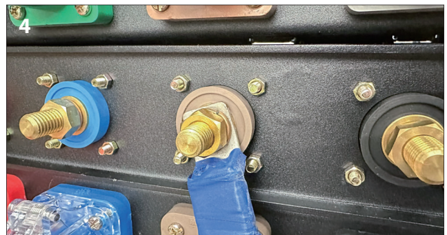
4 Refit the washer and nut onto the threaded post, then tightn to max. of 12N/m
