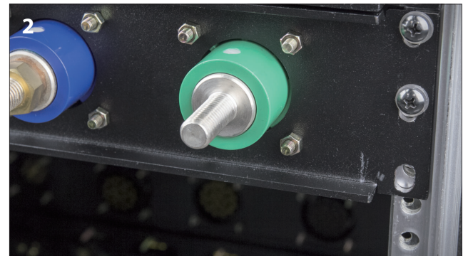
Fit the terminal over the threaded post
